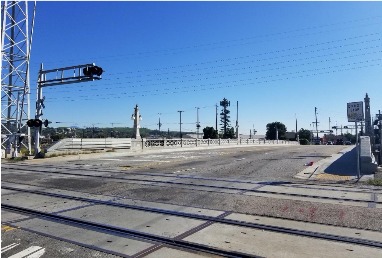
Figure 5-17. North Main Street Bridge from Main Street at the Railroad Tracks (View East)
