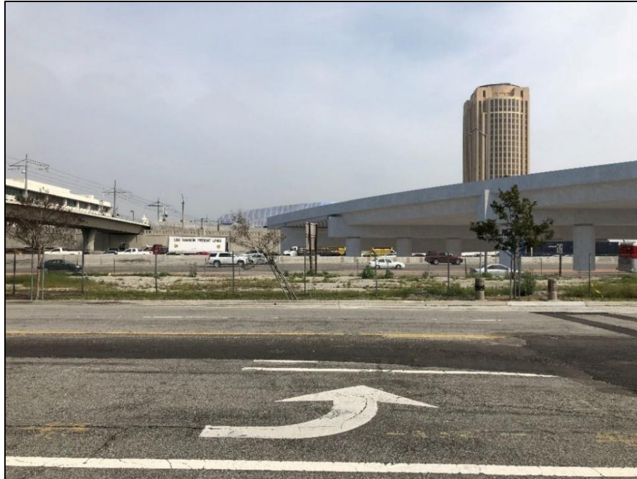
Source: Link US Visual Impact Assessment (Appendix F of this EIS/SEIR)
