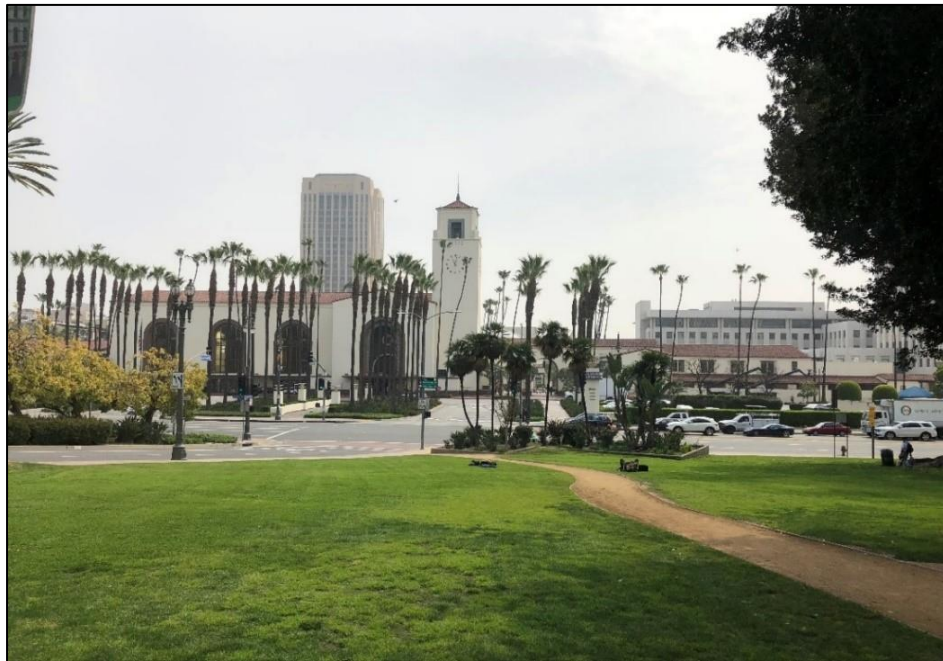
Figure 3.4-36. Key View #4b – LAUS Entrance (view looking east toward LAUS) Existing Conditions
