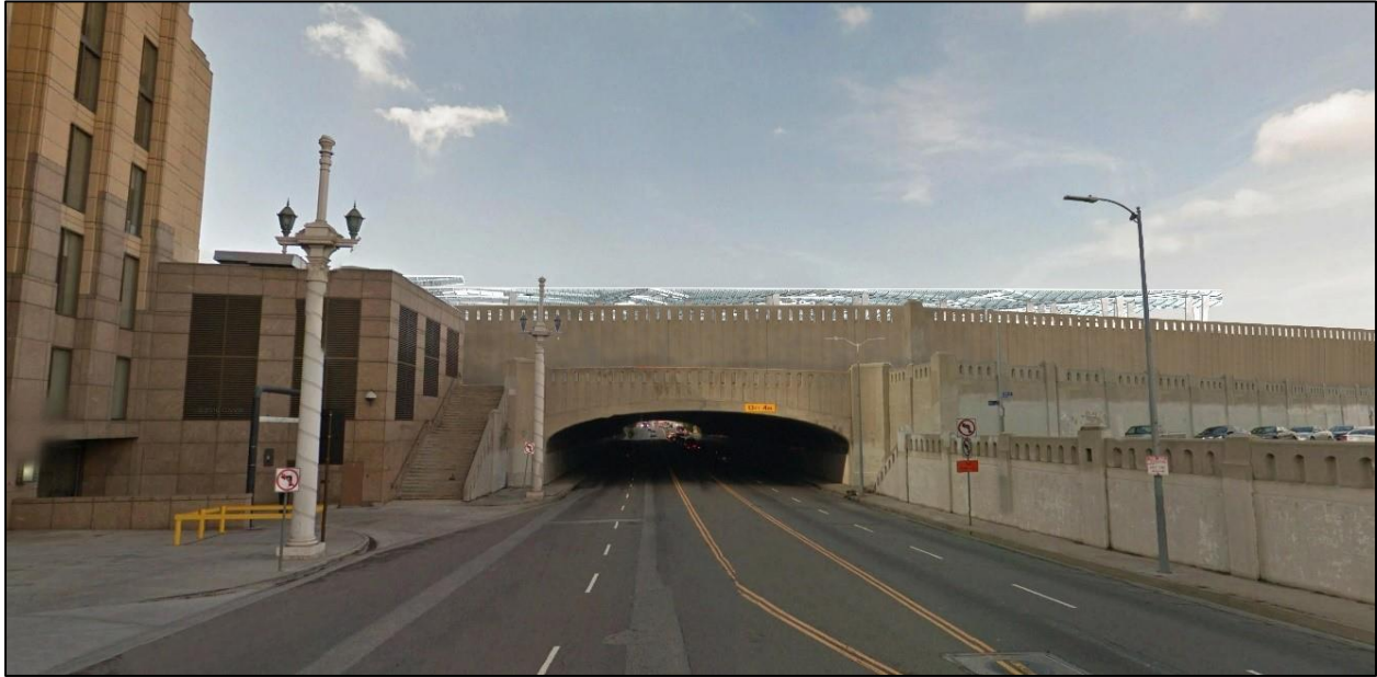
Figure 3.4-31. Key View #3a – Cesar Chavez Avenue Bridge (view looking west toward bridge) Post-Project Conditions with New Bridge and Grand Canopy (Design Option 2)
