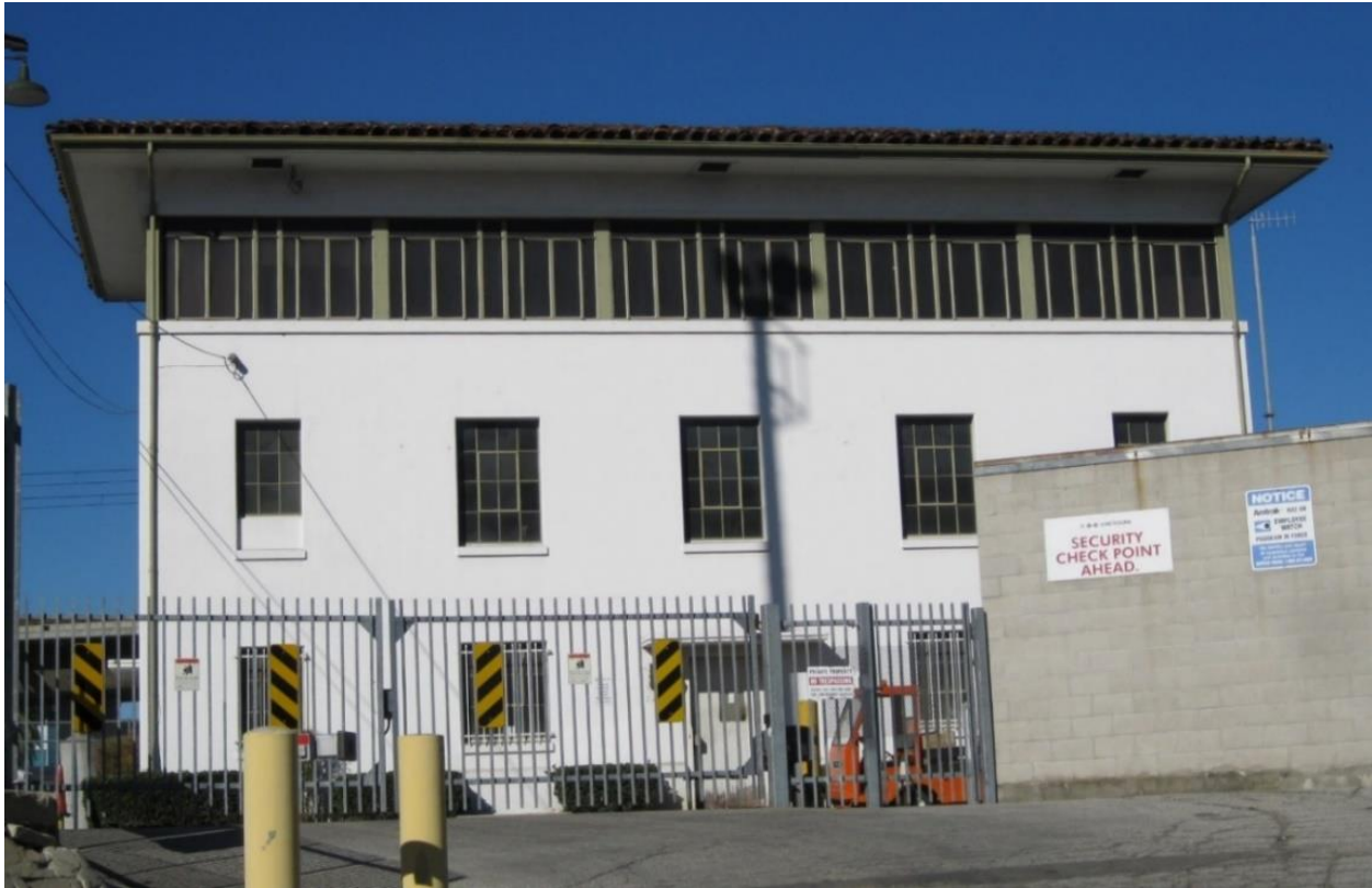
Figure 5-13. Terminal Tower (View Northwest)
