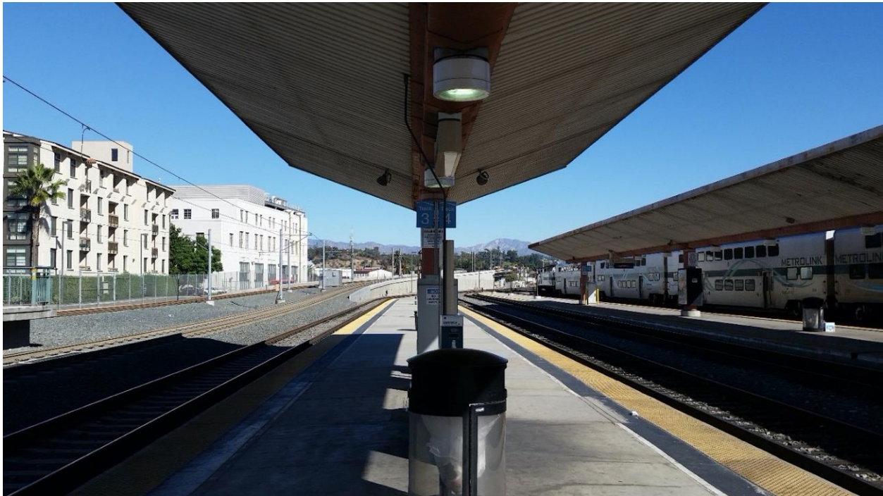
Figure 5-8. Platform and Butterfly Shed Canopies (View North)
