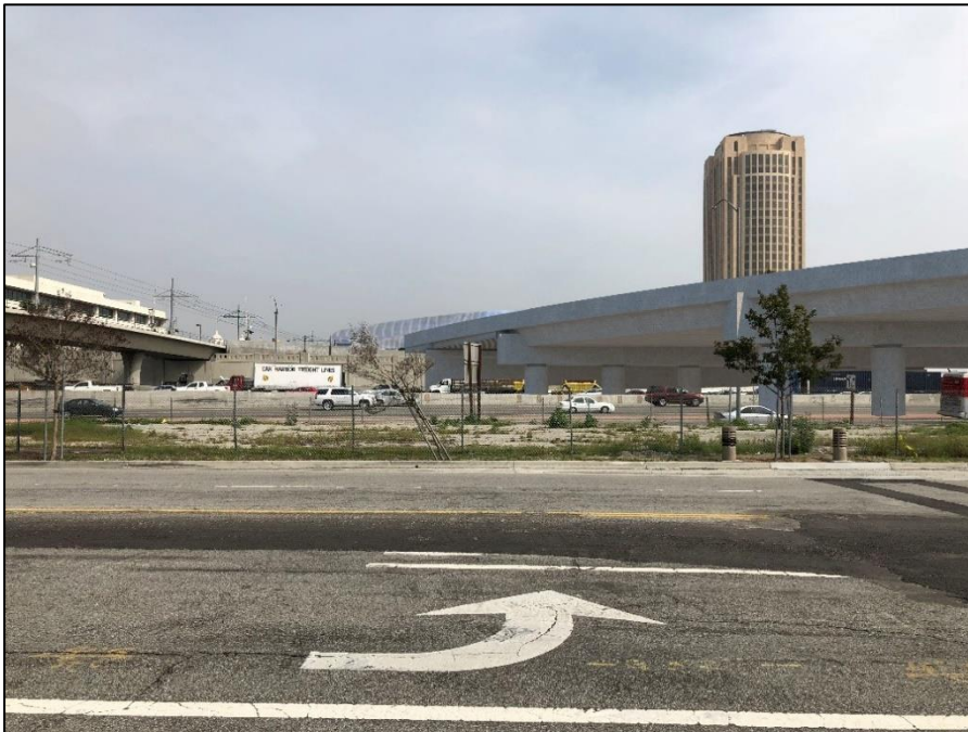
Source: Link US Finding of Effect Report (Appendix M of this EIS/SEIR)
