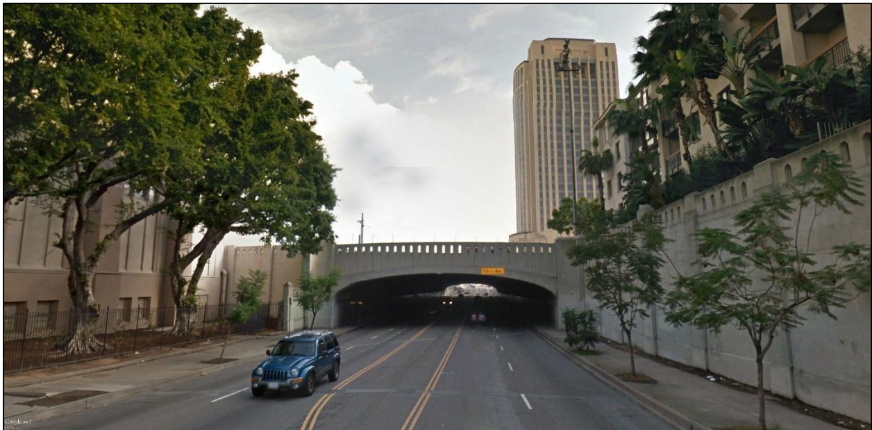
Figure 3.4-32. Key View #3b – Cesar Chavez Avenue (view looking east toward bridge) Existing Conditions
