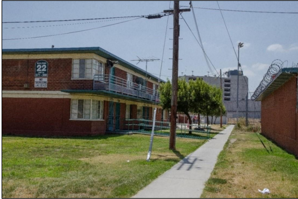
Figure 3.4-4. Key View #1b – William Mead Homes (view looking south from Elmyra Street toward railroad ROW)
